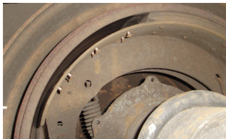
Missing lining block. OOSC, Part II, a.(5)(c)ii / 393.47(a)-U.S.
